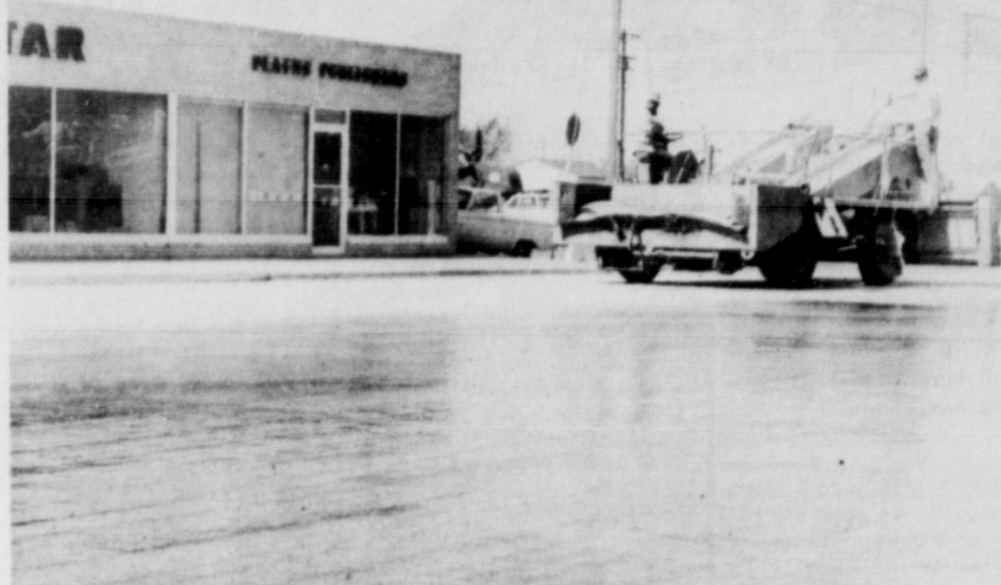
GET SEAL COATING . . . Twenty blocks of Friona streets received seal coats this week. The actual paving was accomplished in one day by Pioneer Pavers of Lubbock.
