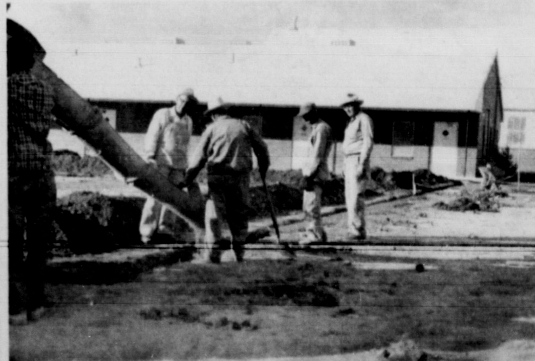
CHURCHES BUILD . . . One of three churches in the city to make building additions is the Calvary Baptist Church, which began construction this week on a new educational wing.
