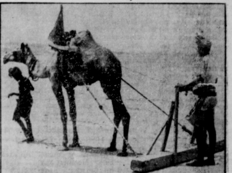
Serenely confident in an age of gasoline engines, an Arab-steered camel helps level an airfield at Aden, Arabia, a base port of Allied supply lines.
