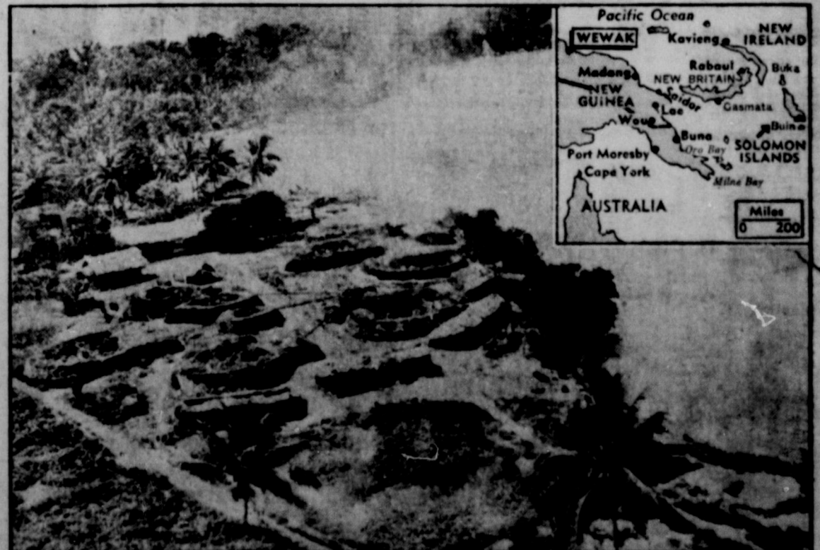
Here are part of the anti-aircraft gun installations protecting Boram airfield at Jap-held Wewak, New Guinea (see map), which Allied flyers must face on numerous bombing attacks. This time the Nips were caught napping, for not one of the guns in the fortified emplacements was in action when a photographer in a palm-topping B-25 Mitchell medium bomber snapped this picture. Madang, another big Jap base, lies between Wewak and the Allied ground forces fighting up the coast past Lae. Another force—American—is at Saldor. (USAAF photo.)
