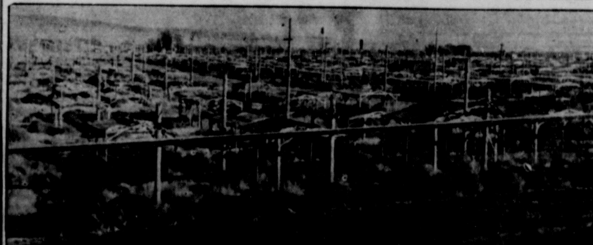
Weeds grow where 80,000 workers and families lived. Only skeleton framework remains of dismantled homes.
