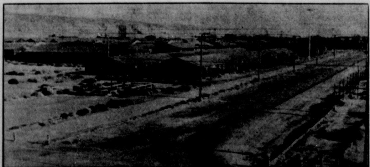
Statesmen wrangle over the atom bomb, and President Truman has stated that we're still making them, but from looks of the engineer works at Hanford, Wash., where a vital part was made, you might think it a dead question. At peak, 45,000 worked in the 631 square mile site. Now coyotes roam there unmolested.
