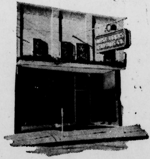
Recently remodeled WTU office at Clarendon
