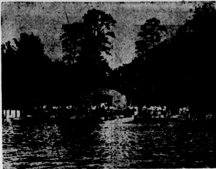
HUNTSVILLE STATE PARK is on a paved park road that leaves U. S. Highway 75 six miles south of Huntsville. The park now has a 300-acre lake behind a dam that was rebuilt last year. The spillway of the original dam was washed out by a heavy flood in 1940. Its replacement was financed by selling timber selectively cut in the park's 2,000-acre forest. During the idle period the lake was expertly managed to get the best fishing, it was opened to fishermen June 1, 1957. Photo by Frank Dobbs, Huntsville.
