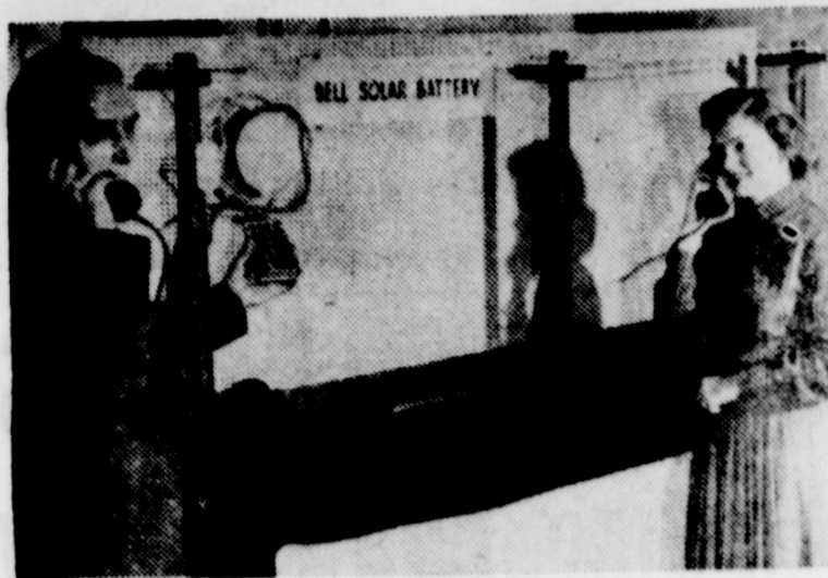
Electrical current to transmit conversation over this demonstration telephone system is furnished from the Bell solar battery which Gerald L. Pearson, one of the co-inventors, is holding under the artificial light. The battery transforms the light into electrical energy.
