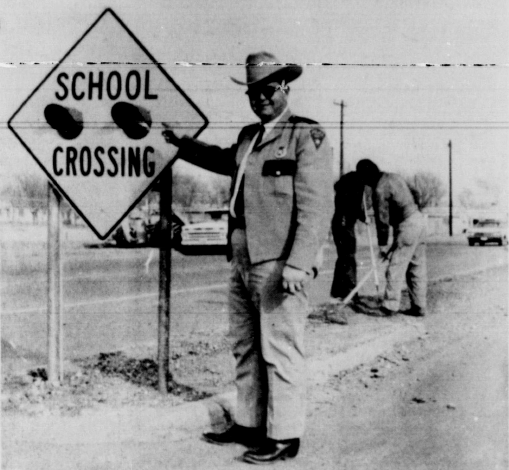
SAFETY MEASURE. . . Friona Chief of Police Travis Clements points to the new flashing signal on Eleventh Street which will be a reminder to motorists passing Friona Junior High School to decrease their speed during school hours. The sign was installed on Tuesday.
