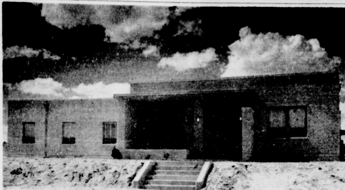
RANKIN HOSPITAL—The doors of the recently-completed Rankin Hospital will be thrown open to the public from 3 to 6 p. m. Sunday in an open house celebration marking the occupancy of the modern medical facilities. First admissions to the new hospital are scheduled for 8:00 a. m. Monday. (Photo by Johnson).
