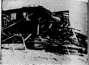
LAS VEGAS, NEV .- This is a "morning after" view of two-story iwelling 3500 feet from A-Bomb last test. Blackened wall ignited but bock waves extinguished flames.
