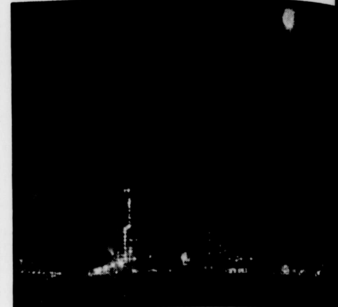
PORT ARTHUR, TEX.—A fitting symbol of fire prevention, 200 ft. refinery flare burns up fire hazards before they start. For wasting gas—as often wrongly supposed—it actually is a safety device. During emergencies it consumes excess gases before they can build up into explosive concentrations; stands 24-hour guard to burn off possibly dangerous fumes. This unusual view of night light at Gulf Oil refinery here was taken in a 10-second exposure at F11 fast panchromatic film.
