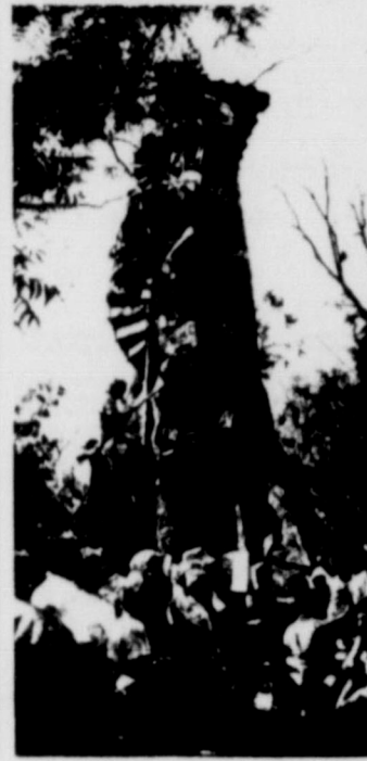
The 44' tall swamp tree slide on Skull Island at Six Flags Over Texas is built around what once was a tire escape at a dormitory at the University of Texas. Guests climb the spiral staircase around the outside of the tree and slide down the long corkscrew-type slide inside.
