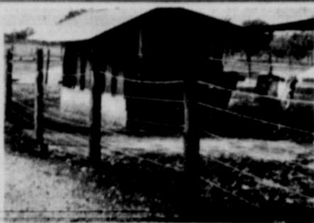
Labor-saving self-feeders at Cattle Feeders, Inc., Goliad, are filled two or three times weekly with 10,000 to 12,000 pounds of mixed feed.
