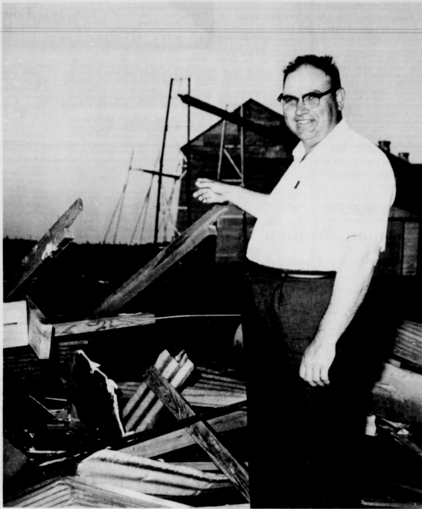
TORNADO DAMAGE. . . James Mabry points to wreckage of a barrack building on the North Lazbuddie Gin property, demolished by a funnel cloud last Saturday. The gin itself,
