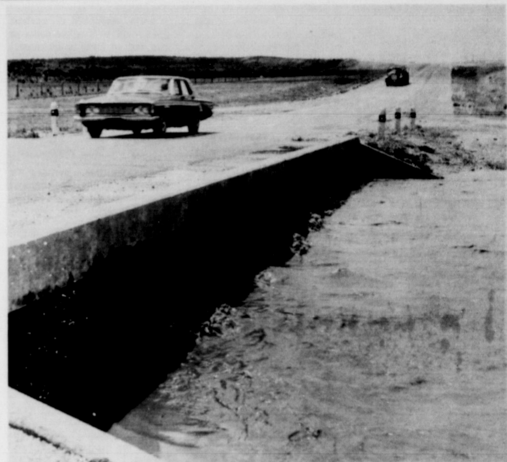
IT WAS RUNNING. . . "Running Water Draw," lived up to its name, as proved in this shot at the bridge south of Friona. The shot was taken on Sunday, showing the water running swiftly near the bottom of the bridge.
