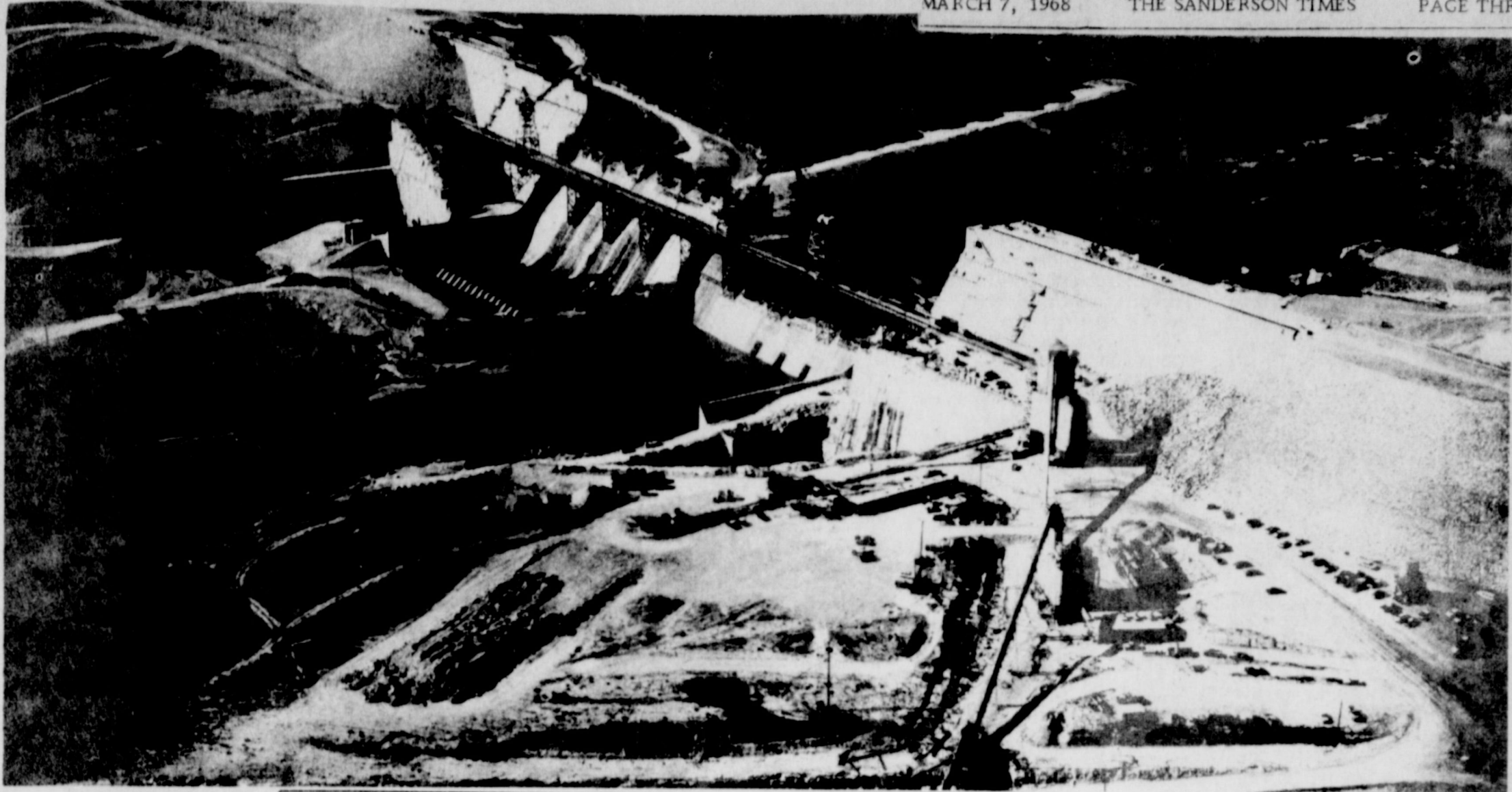
Amistad Dam is nearing the 85% completion mark, according to information received recently. An aerial view of the dam taken January 25, 1968, shows the Mexican side at the right and the U.S. side to the left. The picture is from the Del Rio News Herald.
