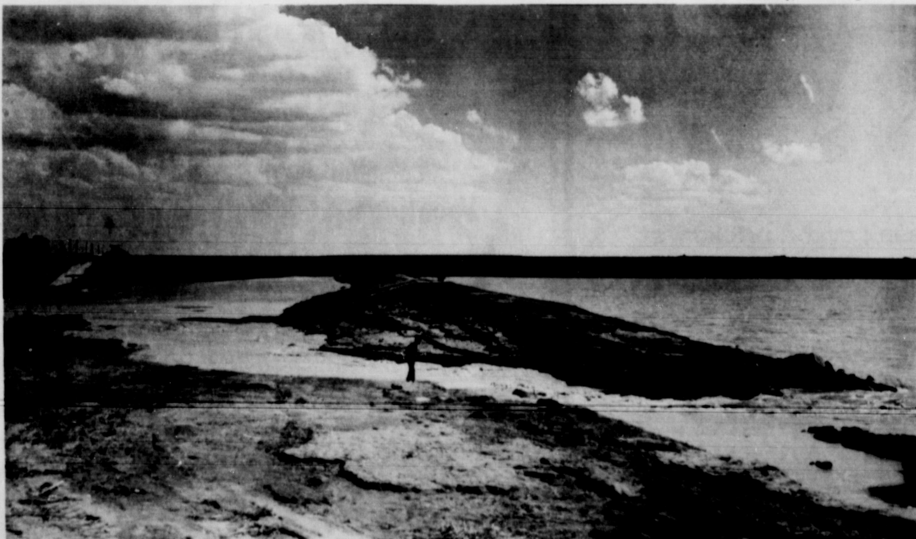
MORE THAN ENOUGH . . . The dam across Frío Draw at Harlan Frye's place east of Friona wasn't tall enough to hold all the water that came down last weekend. The water was running over the spillway Monday and Tuesday. Frye is at-
