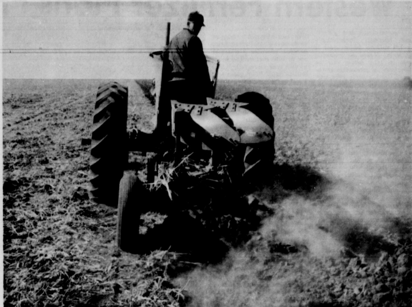
The two-way or "roll-over" plow is utilized to good advantage by many High Plains farmers, especially when they do such fall plowing as is shown above. In the left picture the tractor is headed east. In the right picture it's headed west after the driver has turned around and "rolled" his
