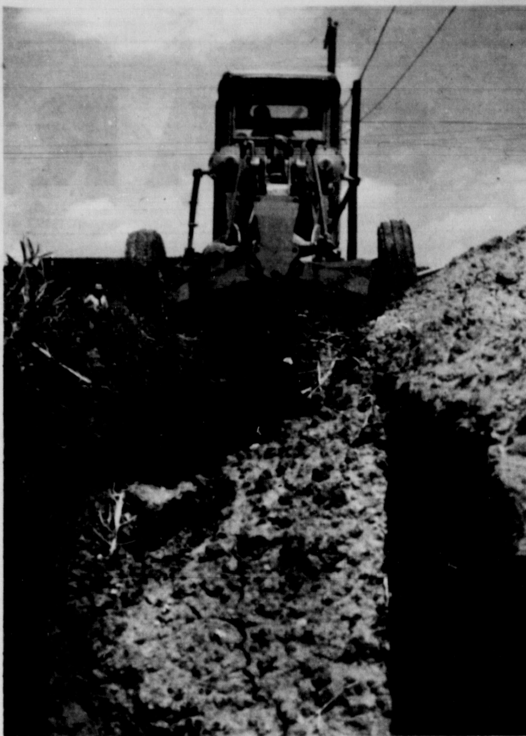
FINISHING TOUCHES . . . City maintainer covers up new water line, completing the installation of a six-inch pipeline in the Staley Addition, expected to give those residents much better water service.
