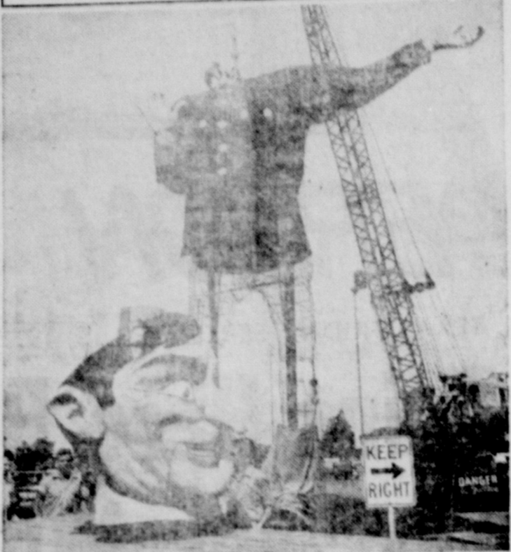
"Big Tex," the towering 52-foot cowboy statue who symbolizes the great State Fair of Texas, is being put together in readiness to welcome some two-and-a-half million visitors to the 1958 exposition, October 4 through 19, in Dallas. It takes a crew of workmen with a 100-foot derrick to put the big boy's head on his shoulders.
