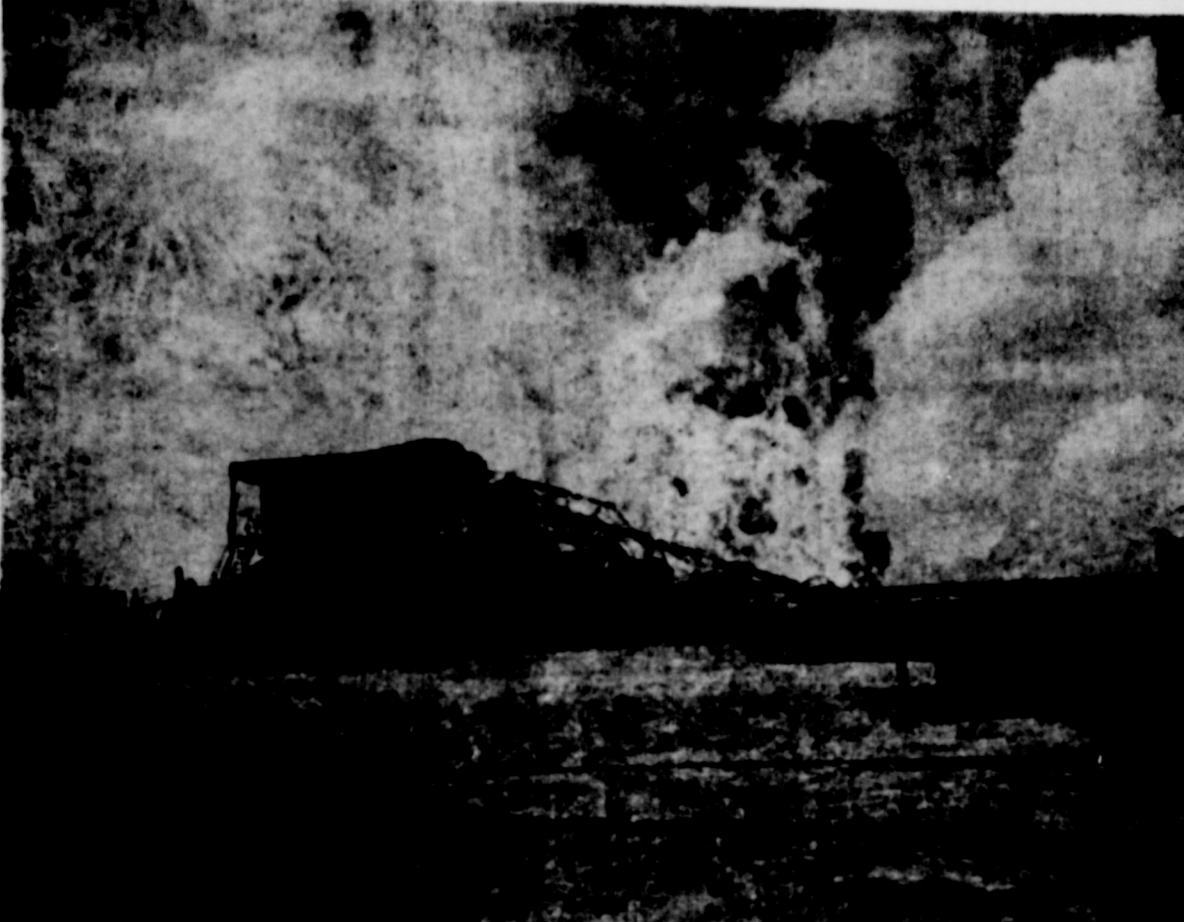
Pictured above is the collapsed derrick at the Brown-Bassett No. 1 being drilled by Magnolia. The picture was taken from the east side of the rig looking to the northwest. All of the debris in the picture was removed prior to extinguishing the blaze. The rig was valued at $450,000 by the Magnolia Co., was a total loss and another is being moved in. —Times photo
