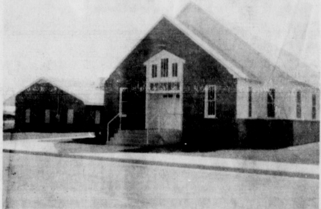
ONE-YEAR OLD THIS WEEK is the Calvary Baptist Church. Shown above are the new facilities which have been constructed during the year the church has been in existence. The sanctuary has a seating capacity of 270 and the educational unit, at left, seats 200.
