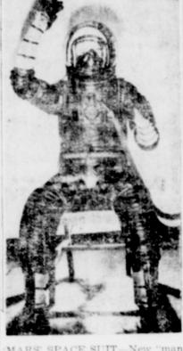
'MARS' SPACE SUIT-New "man from Mars" armor developed for navy rocket or jet aircraft pilots Mr. and Mrs. George Todd or is ground-tested at Washington
