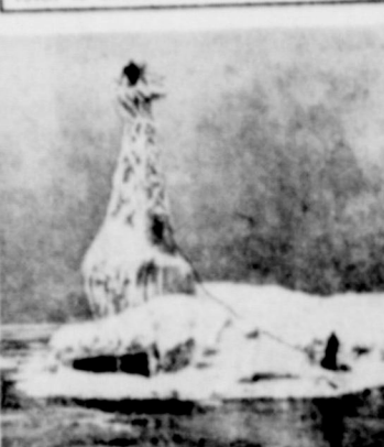
LIGHTHOUSE OBSCURED BY ICE—Tons of solid ice piled up on the 53-foot tower during winter storms on Lake Michigan. Coastguardsmen hack through a thick wall of ice which obscured the navigation light. To seaward a huge field of pack ice stretches to the horizon.
