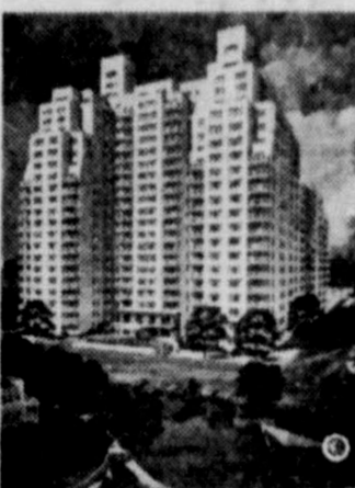
GRACE TOWERS—With its roof-top swimming pool, this 22-story, $10-million luxury apartment house on New York's East Side is Manhattan's latest idea in apartment living.
