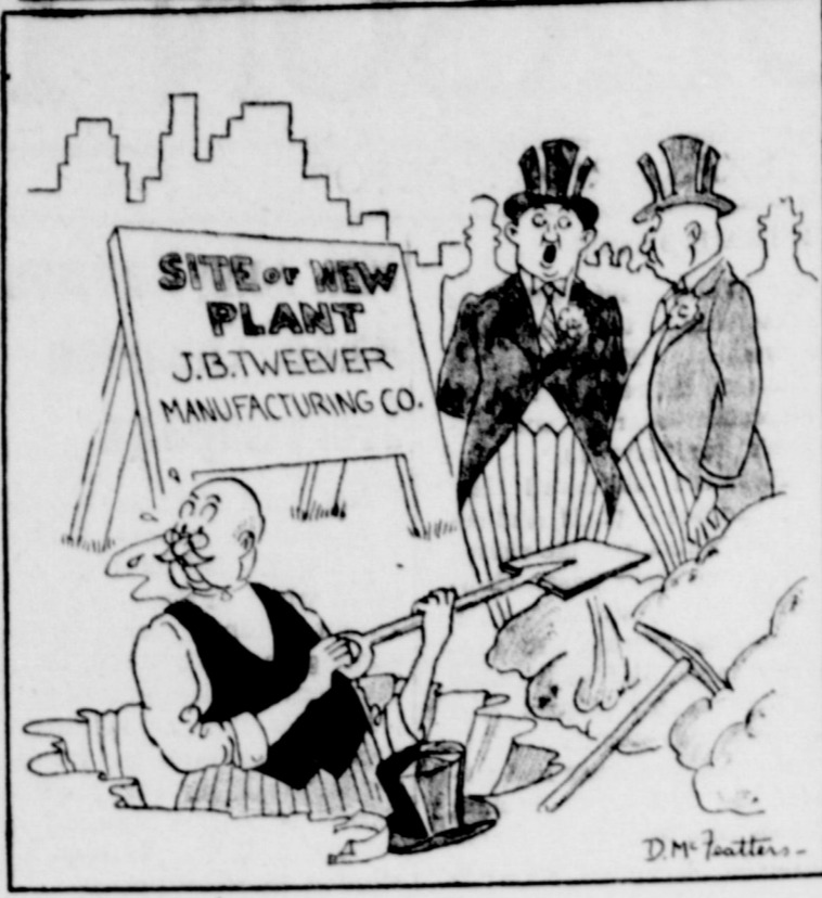
Old "J. B." takes these ground breaking ceremonies very seriously.
