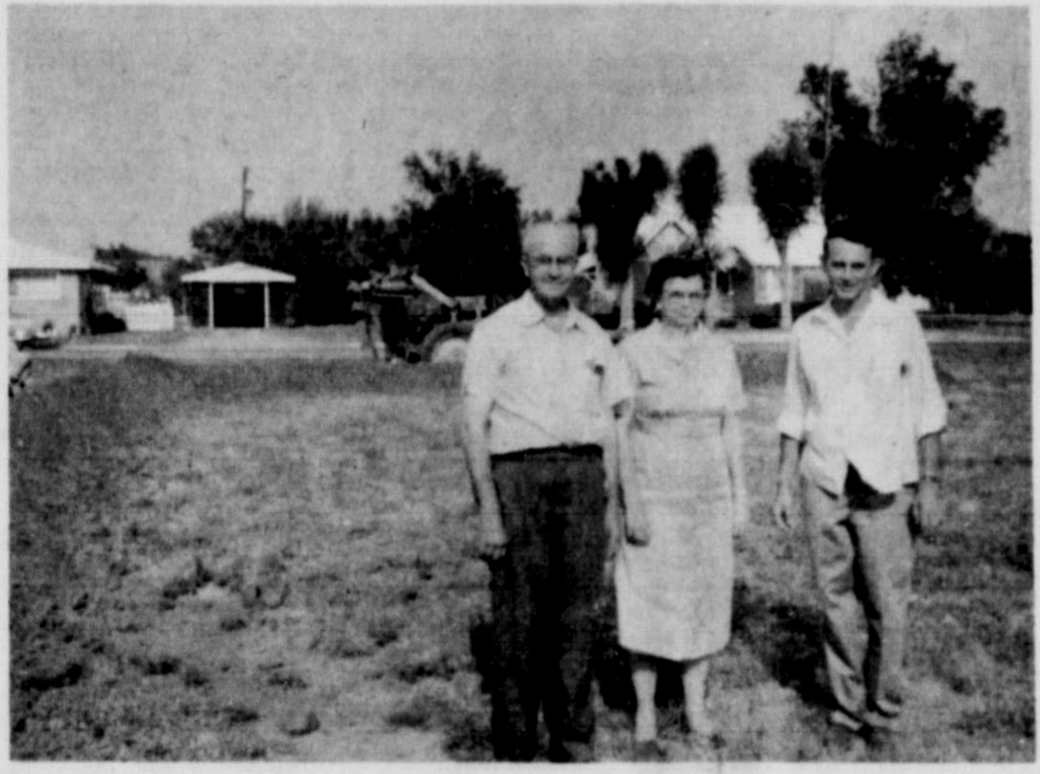
TO OPEN NEW SUPERMARKET--Ed White and his wife and son, Ed Jr., are shown above on the site of their new supermarket on which construction began Tuesday. The new supermarket will also house two more businesses, a ladies shop and an automatic laundry. Robert Schueler is owner of the new building which is being built on the corner of Washington and Ninth Streets.
