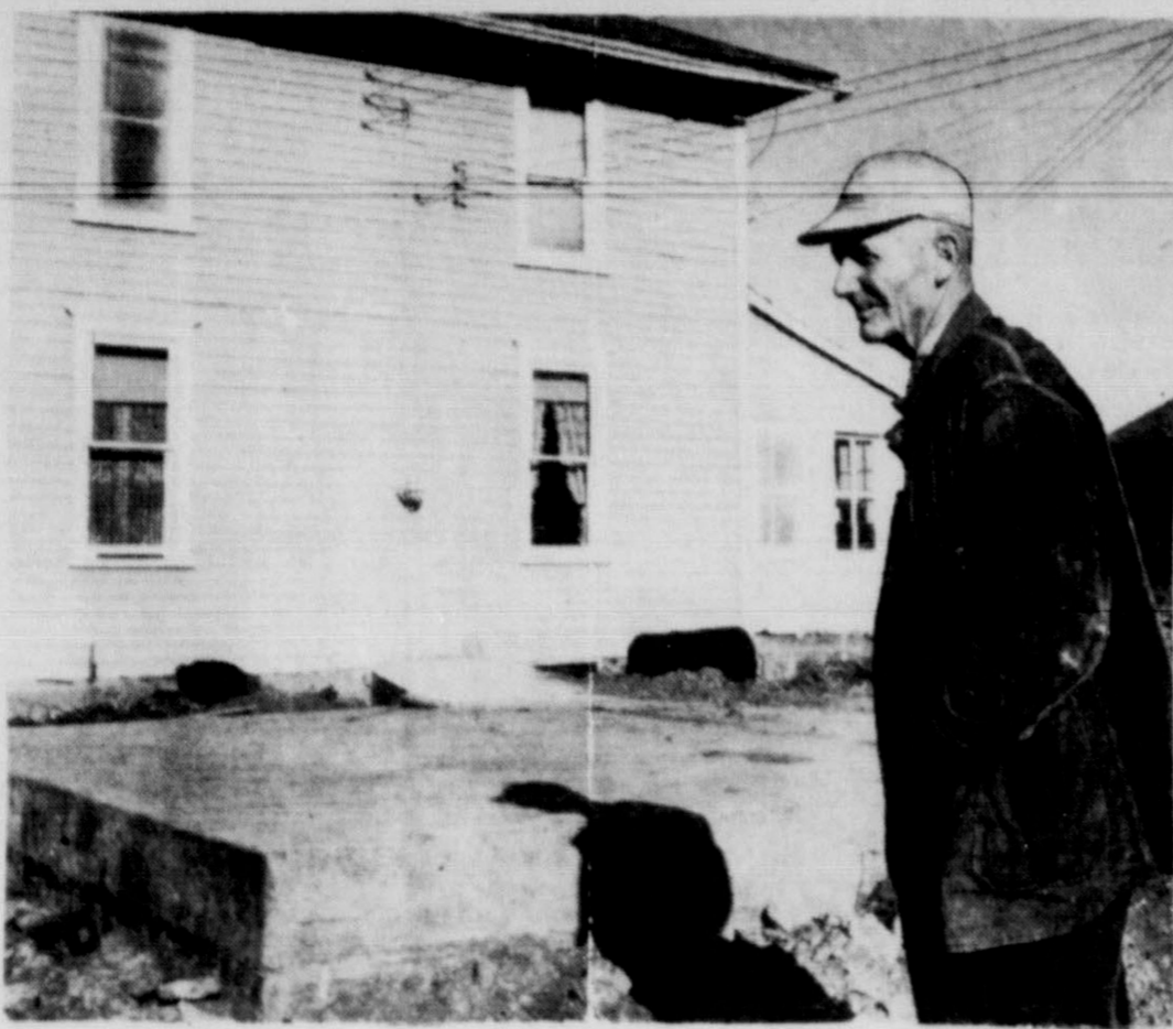
SURVIVAL INSURANCE looks like an ordinary concrete slab at the home of Don S. Trow near Albany, Wis. But beneath the slab is a $1,500 reinforced concrete shelter which the 68-year-old farmer ordered built for himself and his wife. Trow got the shelter plans by writing to Box Home Shelter, Office of Civil and Defense Mobilization, Battle Creek, Mich. (Wisconsin State Journal Photo)
