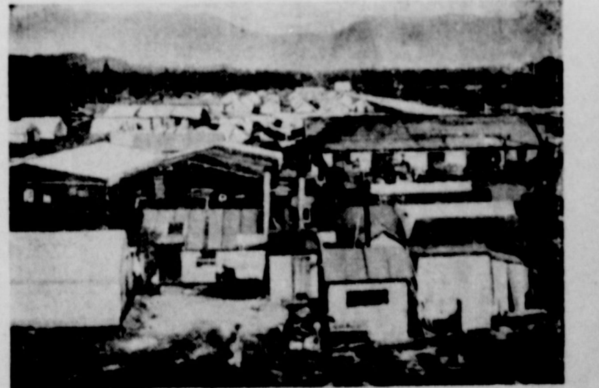
The hardy residents of the state of Minnesota who pulled up stakes and settled on government-owned land in the Matanuska valley, are now settling down for the long, hard Alaskan winter. This picture of the Palmer camp shows the temporary lumber sheds and warehouse. The colonists' tents are in the background. Many homes are springing up.
