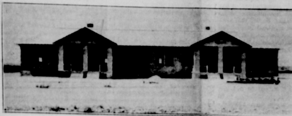
Here is a view of the new barracks recently completed at the Dryden Airport at a cost of $17,000, for the housing of the enlisted personnel of the field and their families. The new quarters were constructed of brick, hollow tile and stucco and are equipped with a
