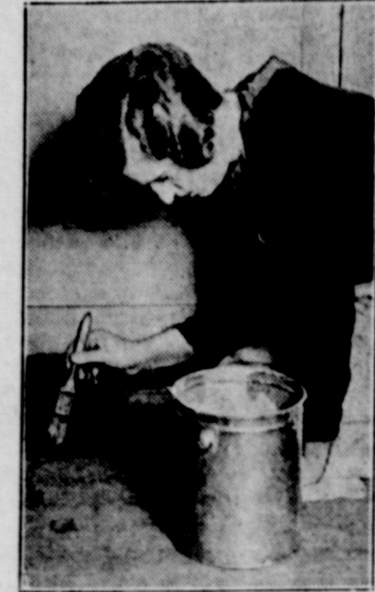
Filling Cracks With Liquid Filler.
