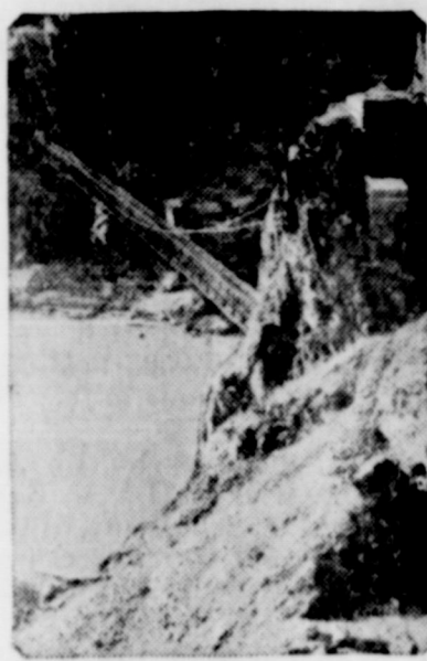
New Steel Footbridge.
