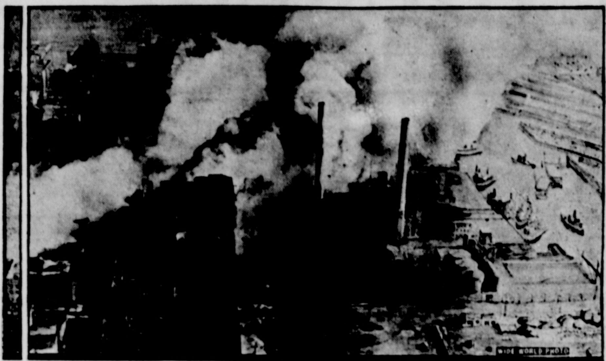
Aerial view of a section of Jersey City, N. J., covered by a pall of smoke from the fire which swept two square blocks, causing property loss of at least $1,500,000. Not many hours later a second conflagration swept the Jersey City waterfront.
