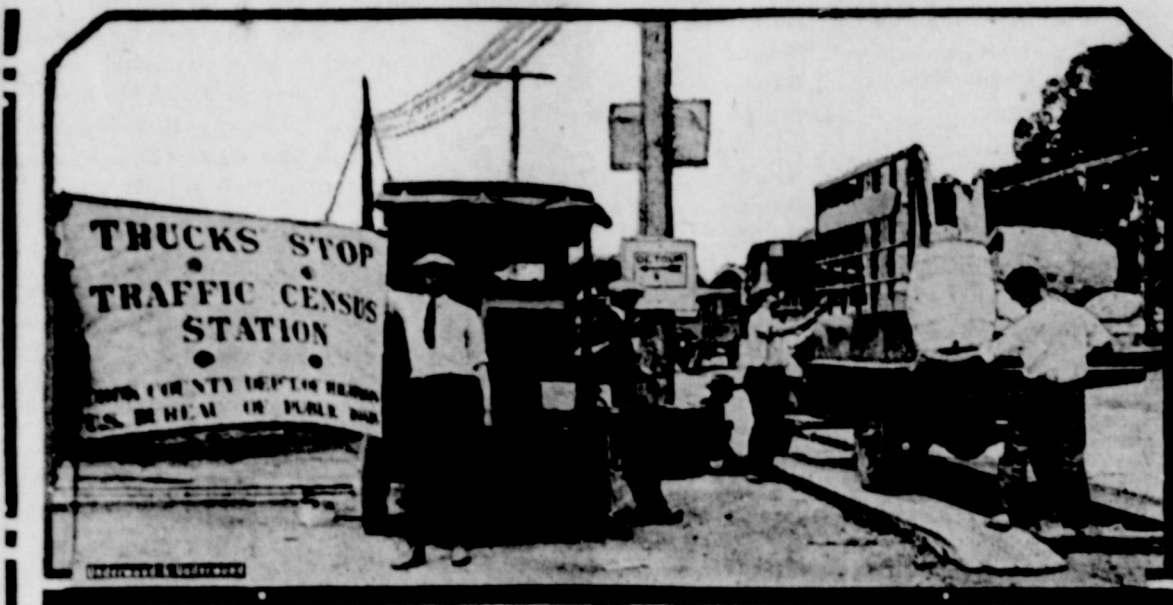
Government and county investigators are making a survey of the roads of Cook county, Ill. With the information obtained they plan to base specifications for more serviceable highways throughout the United States. Picture shows investigators weighing and examining a truck.
