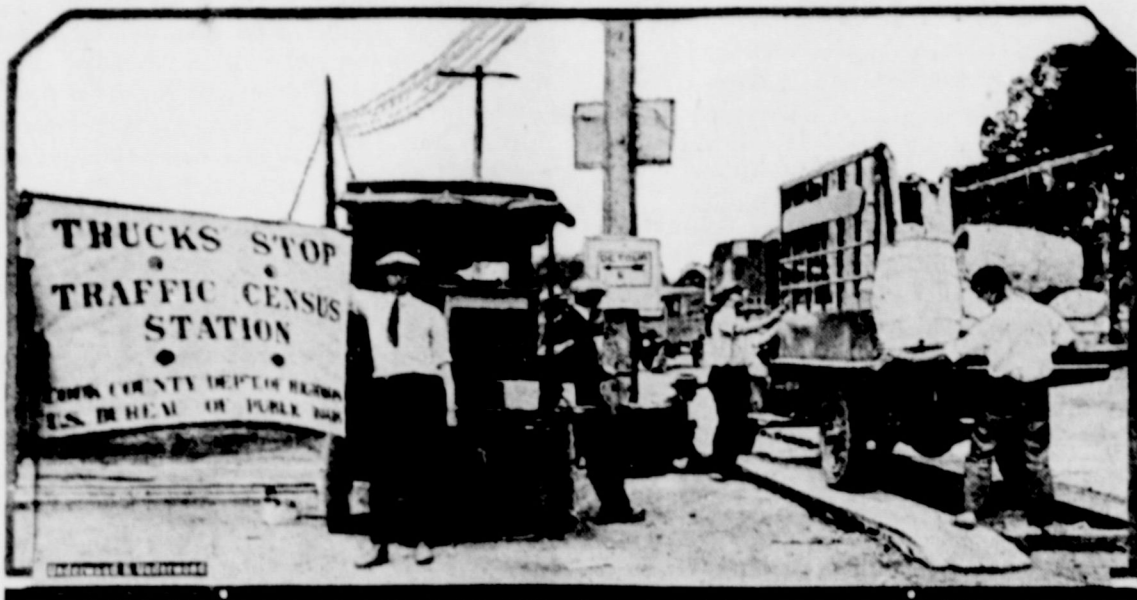
Government and county investigators are making a survey of the roads of Cook county, Ill. With the information obtained they plan to base specifications for more serviceable highways throughout the United States. Picture shows investigators weighing and examining a truck.
