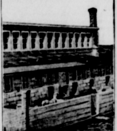
Swine house Made of Concrete Blocks.
