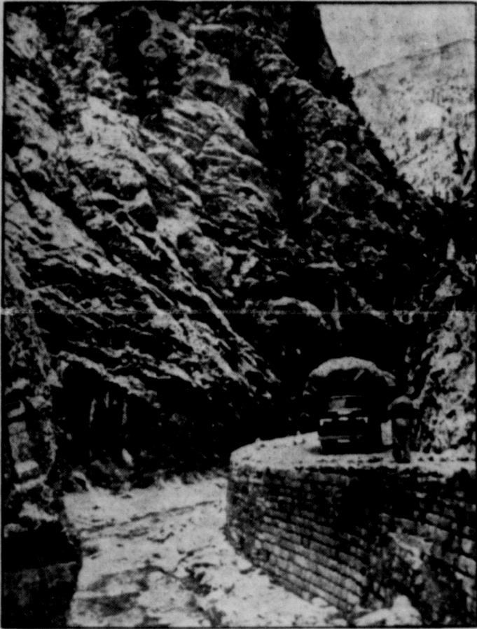
This rugged, narrow road through the Toros mountains in Turkey is typical of that country's highway system. The United States has granted $5,000,000 and the use of U. S. technical experts and equipment to the Turkish government to help in a 10-year program of highway reconstruction. This is Gulek Pass, the route over which Alexander the Great made his way through the mountains to conquer the Middle East.
