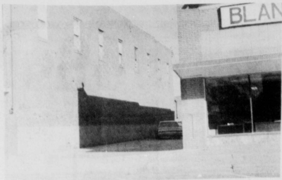
NEW PARKING LOT AND drive way entrance has been completed between Blanco Offset Printing and Williams Meat Market on the north side of the square. The new concrete replaces weedy lot and Blanco's customers can load out of the west door of the warehouse instead of the alley. (Staff Photo)
