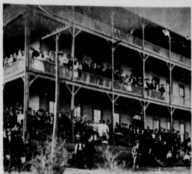
UNION STOCK YARDS, 1890s STYLE—This frame structure housed the San Antonio Union Stock Yards until 1938. That year, it was replaced with the present livestock exchange building which houses the Federal-State Livestock Market News Service offices. This September, the Service celebrates forty years of providing accurate market news to Texas farmers and ranchers, Agriculture Commissioner John C. White said.
