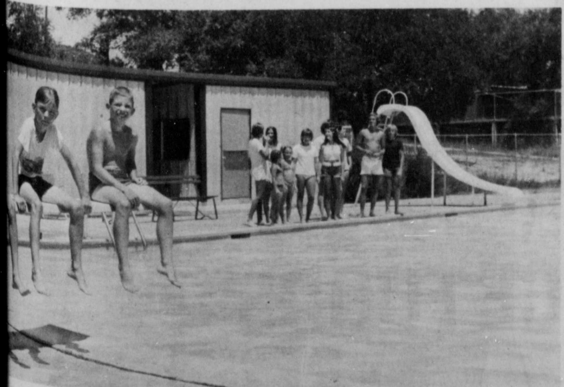
COUNTRY CLUB SWIMMING POOL gets a new bath house which is just about (Staff Photo)
