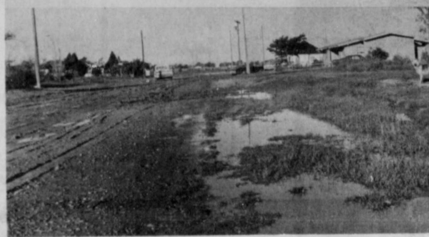
DELLA PLAINS AREA, NO GRADING, NO DRAINAGE
