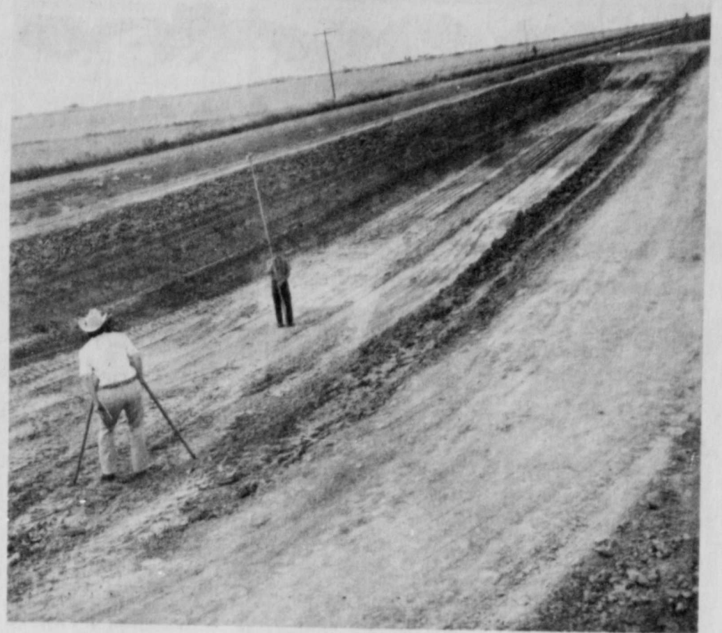
SCS PERSONNEL Fay Gooch and Layton Koch check out tailwater pit on the Connie Bearden farm about 2 miles west of Floydada. The tailwater recovery system will return runoff irrigation water back into the irrigation system to be re-used.
