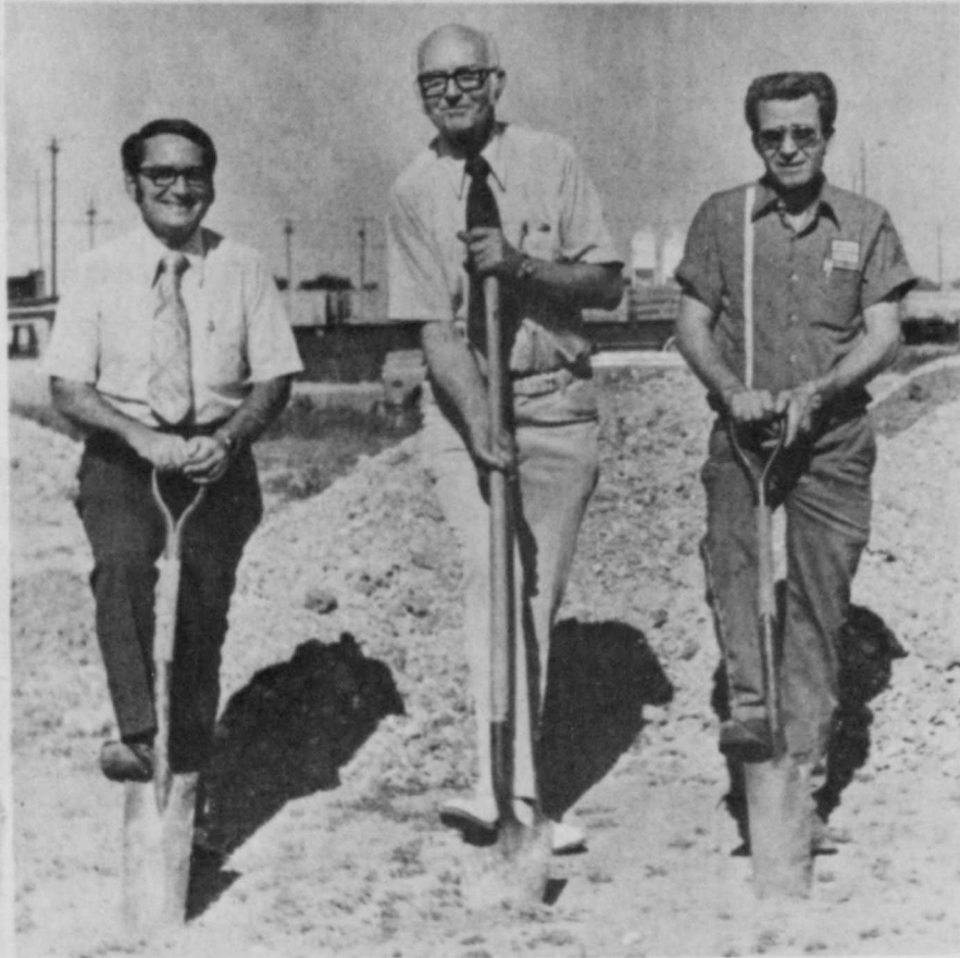
BREAKING GROUND for new fire department building (l to r) Bill Feuerbacher, Mayor Parnell Powell and fire chief Billy Marquis. (Staff Photo by Brad)
