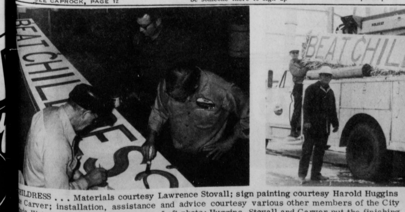
CHILDRESS... Materials courtesy Lawrence Stovall; sign painting courtesy Harold Huggins; Carver; installation, assistance and advice courtesy various other members of the City Water, Power and Light crew. Left photo: Huggins, Stovall and Carver put the finishing
