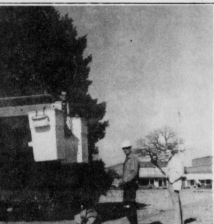
CHRISTMAS DECORATIONS GO UP... Utility-company workmen light the "Christmas Tree" on the court house square in Floydada. They also installed about 40 scroll-type light-pole decorations in the city. (Staff Photo)
