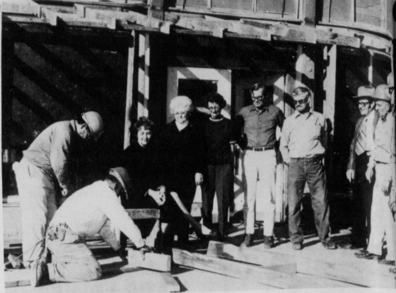
WORK STARTED ON MUSEUM BUILDING . . . Green Thumb workers and local citizens gathered for the laying of the western front to museum building on the north side of the square. Pictured left to right: Cisco Granados, Casimiro Nava, Mrs. Q.D. Williams, Mrs. Alma Holmes, Mrs. (Mrs.) Ted Bell, Eli Neff, Robert L. Smith, Allen Rendon and H.O. Ginn.
