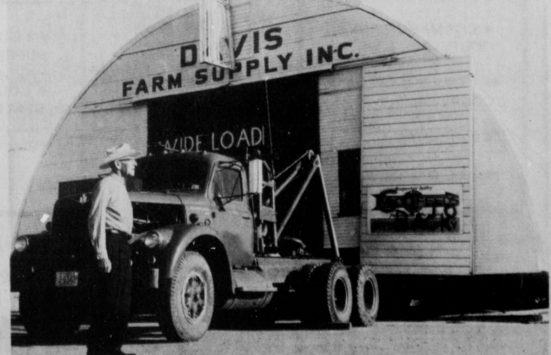
THE FIRST FARM CHEMICAL BUILDING . . . in the county is loaded and ready to be moved to make room for a modern building. Harry Morckel, who opened the business in 1950, takes a last look at the building in its original location. (Staff Photo)
