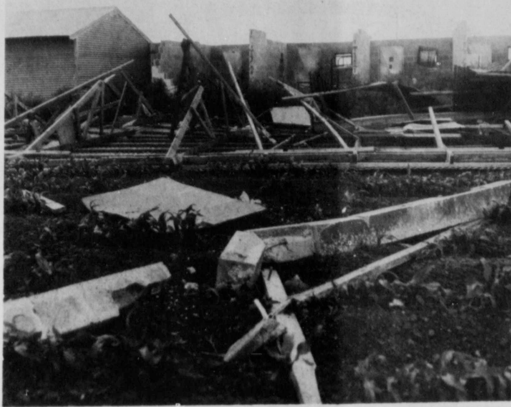
FREAK WIND . . . lifted the roof off this barracks building at Brown Gin south of Floydada Thursday morning, also taking off the back wall (shown) and scattering the wreckage over a field north of the building. (Staff Photo)
