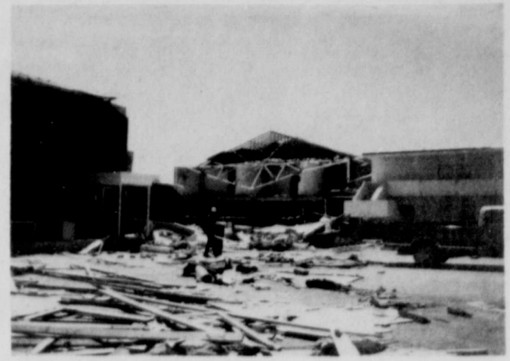
FIRST BAPTIST CHURCH in Portland, Texas, completely destroyed by Hurricane Celia.
