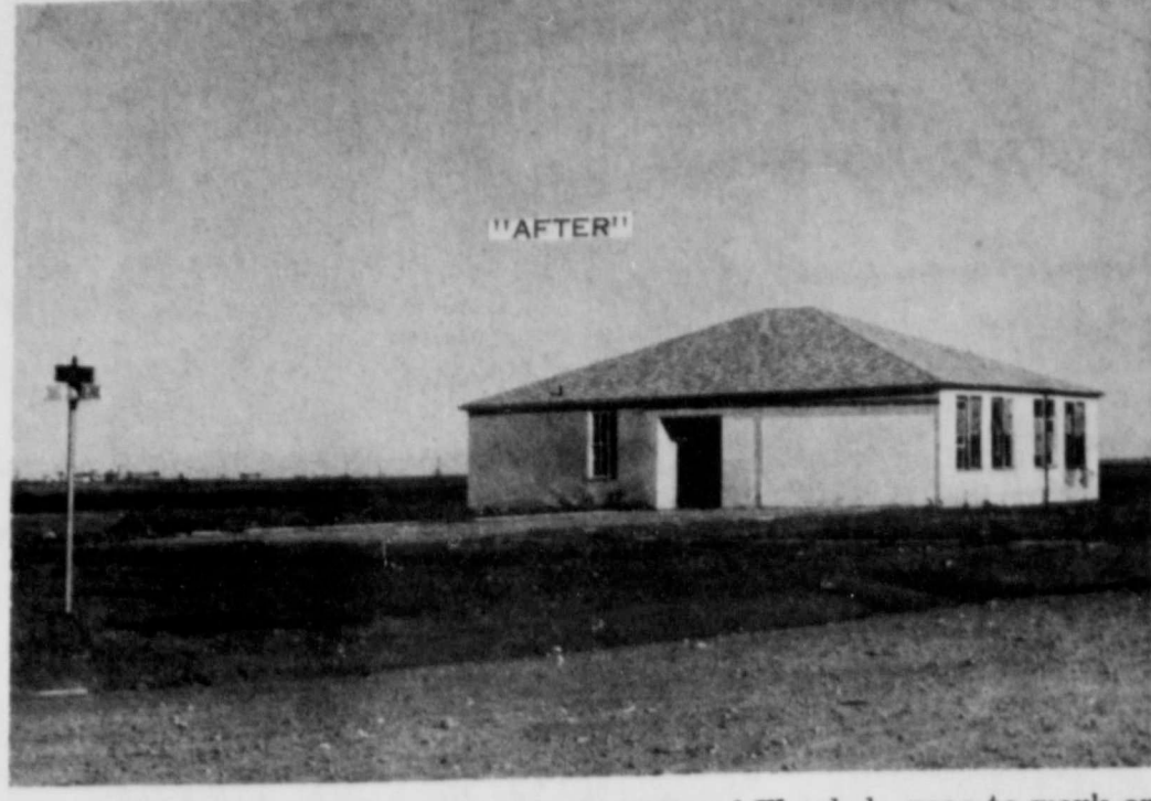
park area to show what happens when the City of Floydada goes to work on cleaning up an area...the "before and after". (Staff Photo)
