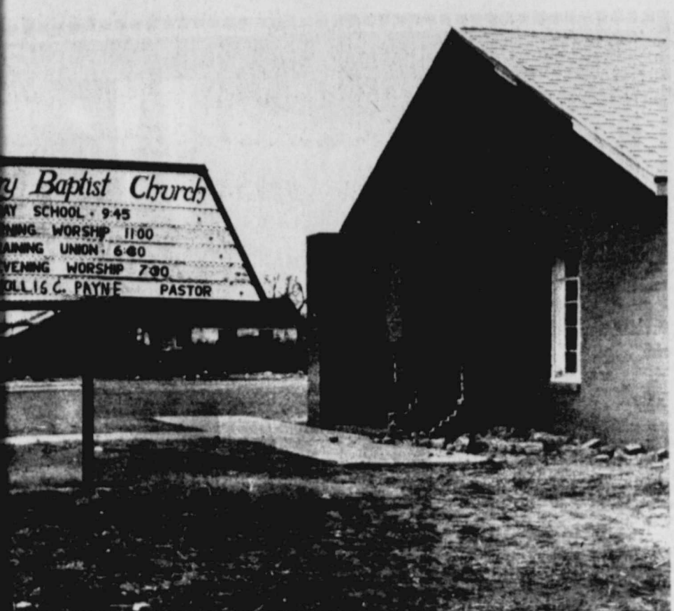
CRASHES INTO CHURCH... Danny Daniels of Blanco Community, lost control of his car and crashed into the entrance of the Calvary Baptist Church at 1:30 a.m., January 1. (Staff Photo)
