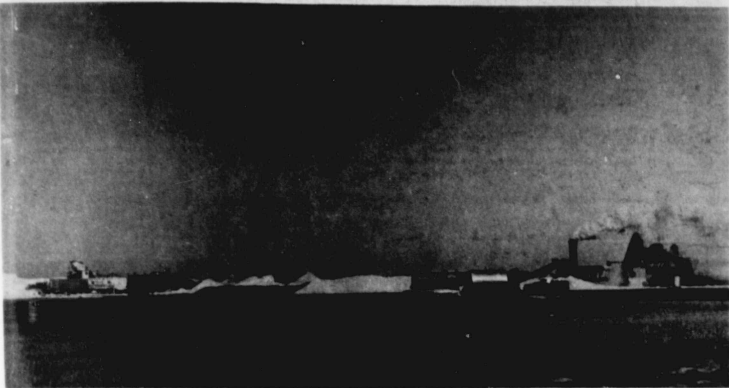
NEW FLOYDADA INDUSTRY is pictured above. . . . it's Gifford - Terrell of Amarillo at the Maud Hollums caliche pit about five miles north of Floydada. Several men are employed in crushing the caliche, operating the hot mix plant, trucking butane, sand and petroleum into the plant and caliche and hot mix out to the road building job east of Floydada. It is reported to be the best grade of caliche rock in this area. (Staff Photo).
